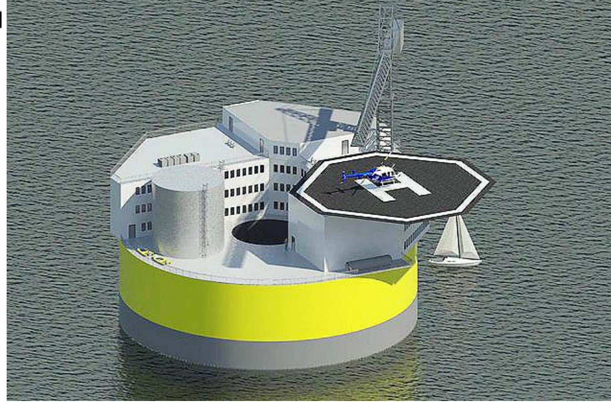
This illustration shows a possible configuration of a floating offshore nuclear plant, based on design work by Jacopo Buongiorno and others at MIT's Department of Nuclear Science and Engineering. Like offshore oil drilling platforms, the structure would include living quarters and a helipad for transportation to the site.
